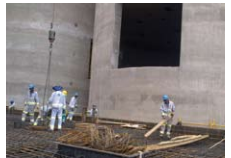
Construction work at the conditioner building
