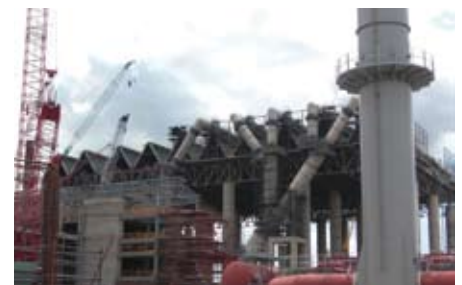
Medupi is the worldwide largest dry-cooled power station
