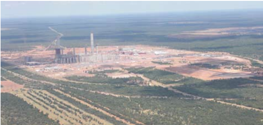
View of Medupi power station, Lephale, in South Africa
