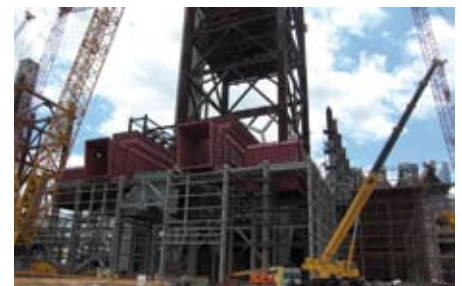
Duct work under construction
