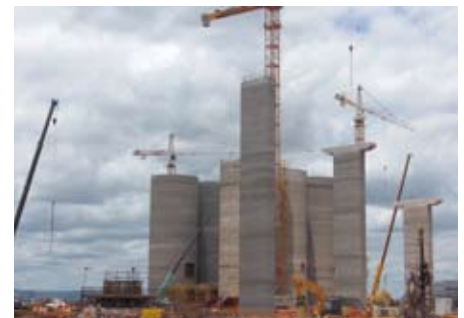
Fly ash silos under construction
